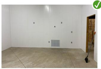
FRP Panels. Installed to the bottom of drywall. Flat and secured, not wavy, cracked, or uneven.
